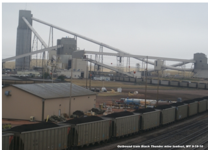
Outbound train Black Thunder mine loadout, WY 9-18-10
