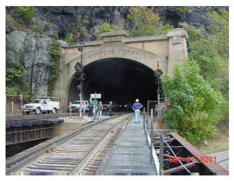
Five vehicle Hi-Rail field check trip on CSX from Weverton, MD to Martainsburg, WV stops at the Harpers Ferry Tunnel to check for new signal locations. Vehicles are on the mainline, track in foregroundis the Shenandoah Sub. Photo by Rick Schroeder
