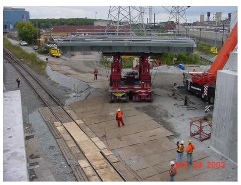
So you want to move a bridge! On September 28 Kiewit Western hired Mammoet Systems to move in the two bridge structures at the Metra bridge crossing over CSX and NS at Riverdale. Shutdown started at 7 PM on the 27th, at 2 PM the contractor started moving the bridge from the parking lot and set in place over CSX, ready for track, around 5 PM on the 28th. NS was finished at 2 AM the following morning. Photo by R. Schroeder
