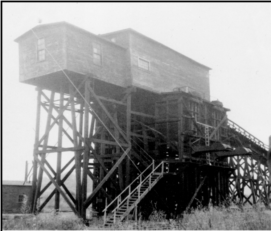
NYC Coal Dock at Lyons Yard, Westville (Belgium) II. On August 10, 1955 a 15-year old Hank Sherwood and friend ventured into Lyons Yard. Hank photographed the 200-ton wooden coal dock used to fuel locomotives. This dock had a 20% grade and the back of the building is the winch house used to winch up the loaded hopper cars. It was built in 1907 at a cost of $10,300. Photo by Hank Sherwood, Danville Junction Chapter collection.
