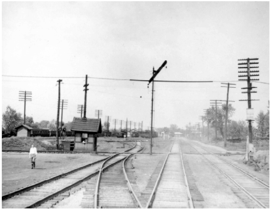
The Barringer photo, taken in the late 1930's, is from the rear platform on a westbound Wabash train. This is Danville Junction, the same location as the cover photo. The P&E is the line crossing left to right by the shanty. The C&EI "City Main" is on the left and the "Westville Branch" is the curve track toward the photographer. The crossing was protected by a "target" signal. The arm is up for a "highball" for the Wabash. When this crossing was electrically interlocked it was transferred to the "tower" at the mainline crossing, some 1/4 mile behind in this photo. Photo by Barringer, from the collection of the DJC.
