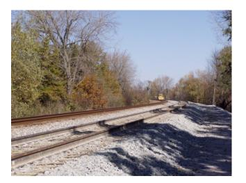
To finish out the series on the #2 main extension project, here are three images. *At left* on 11-4-07, the ballast regulator was finishing up the last brooming work on the new track behind my house.
