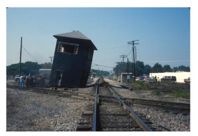
I posted this photo on a tower Facebook site last month. The date is August 24, 1994. We had completed the construction and tie in of the new track alignment at Iles interlocking in Springfield and it was finally time to remove the tower. The asbestos singles had been removed, the Wabash line was out of service and the tower was pulled over.
