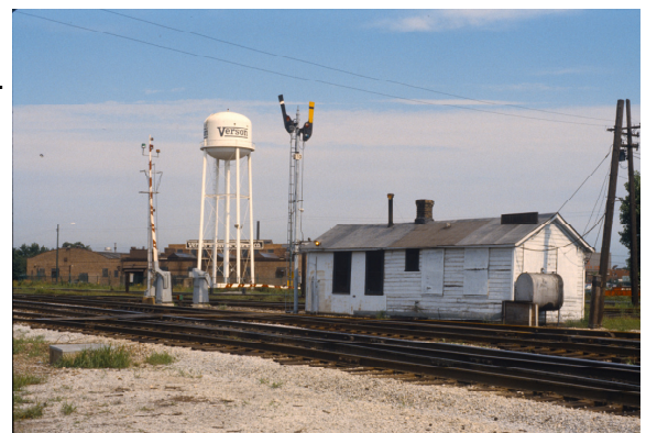
Pullman Jct, a system of blades, gates and flashing lights controlled the NKP/C&WI and Rock Island Crossing at Stoney Island. R Schroeder 8-15-79
